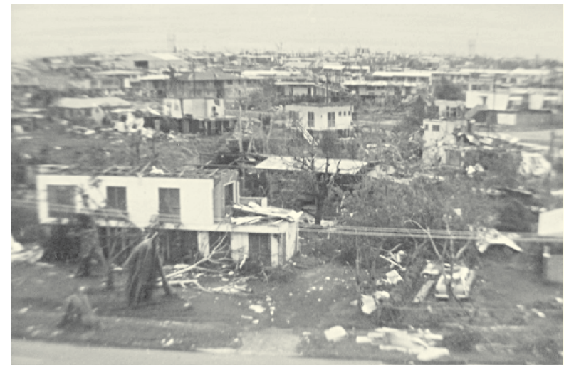
[Billbee, Damaged houses after the passage of Cyclone Tracy on Christmas day 1974 in Darwin, Australia , 2007. Source: Wikimedia Commons]
